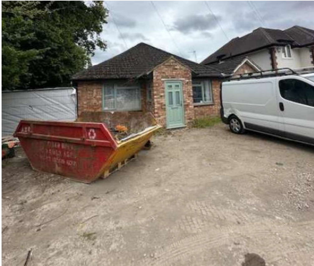
Figure 2: Photo of the Application Property from the street
